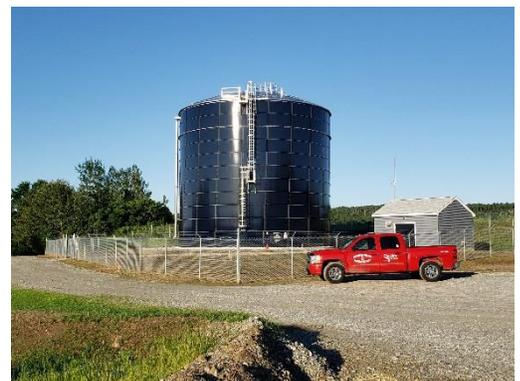
June 2019 – The new 1MG glass-fused-to-steel water storage tank goes on-line. It is 59' wide and 51' tall. Treated water is pumped into the tank from the Pinnacle Pond area. The tank feeds the water into the Village by gravity.
