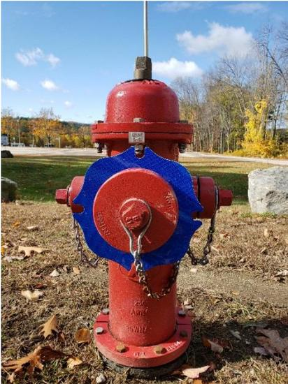
Example of a newly tested and marked hydrant at Donati Park. Blue indicates estimated flows >1,500 GPM at 20 PSI. Markers are reflective to improve nighttime emergency visibility.
